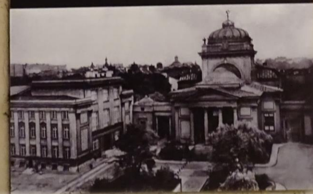
Fragments of Columns from the Interior of the Great Synagogue of Tłomackie Street, 1876-1878
