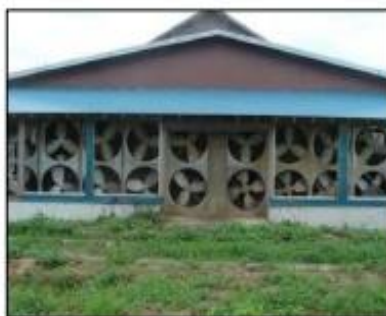
↑牛舎壁面の換気扇
