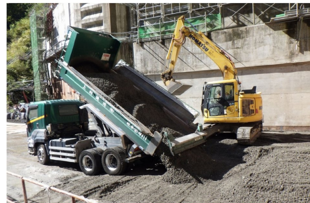
減勢工RCD施工
